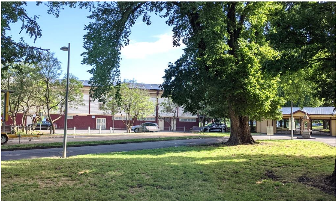
Figure 13 Service area beyond the north elevation of 1888 Grandstand; the timber entrance pavilion is to the right of the image, Bocce Courts (gravelled area) to centre
