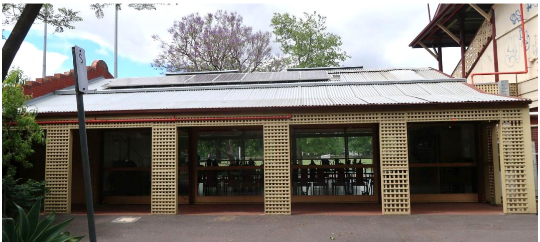
Figure 11 North elevation of community room
