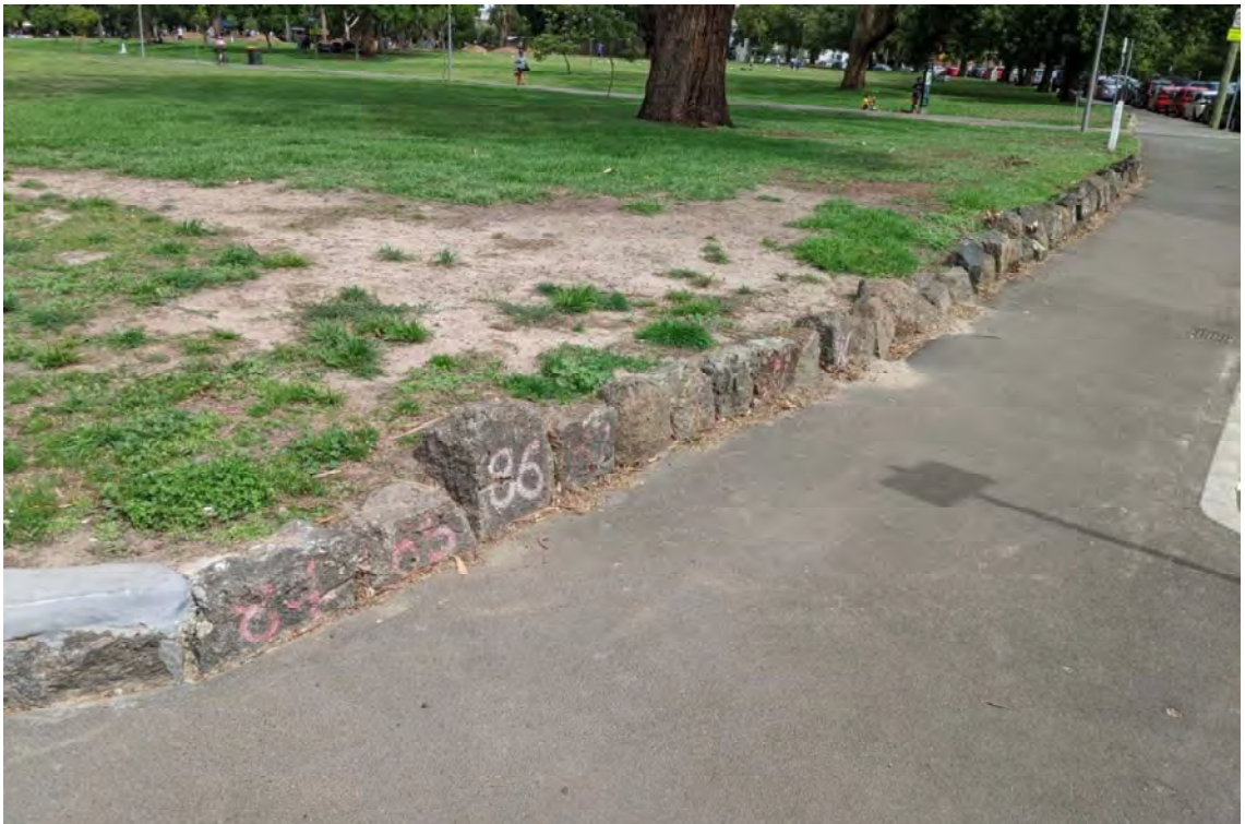
Figure 158 Crenelated bluestone edge to section of Alfred Crescent adjacent to the former railway corridor
