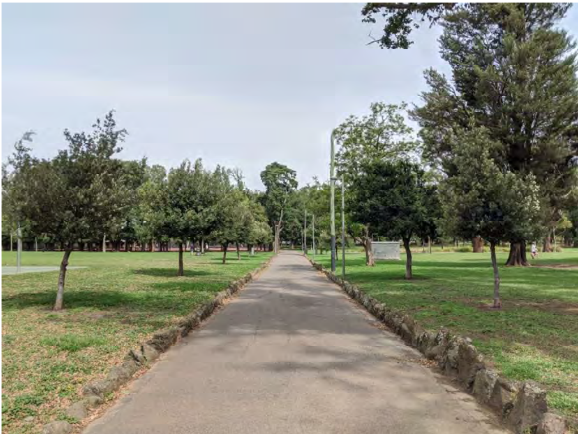
Figure 87 Example of bluestone rubble edging; this form of edging is seen in photographs from the 1920s-1940s, and in many cases served to provide a front edge to garden beds and shrubberies, now removed
