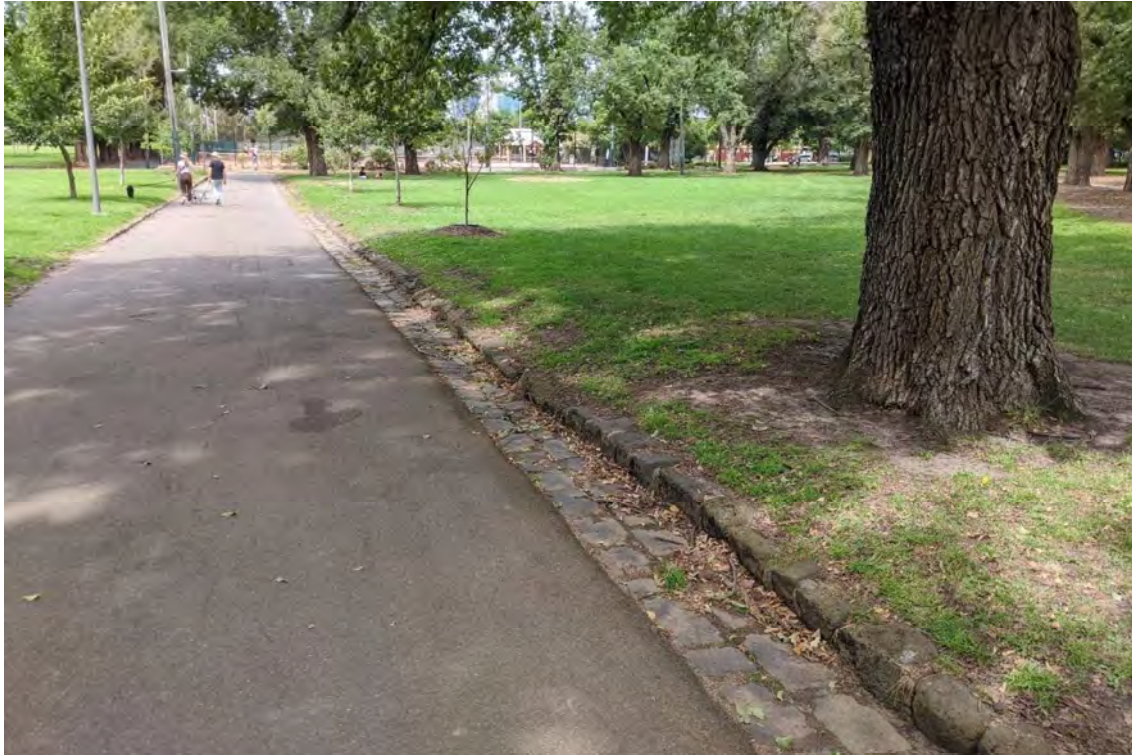
Figure 90 Bluestone channel and edge kerb; this feature appears from aerial photography to have been installed on Avenue A between 1951 and 1969
