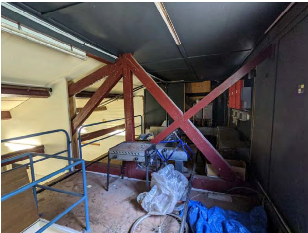
Figure 44 View of the mezzanine area showing the section open to the ground floor, partial enclosure of the truss and modern lining to wall and ceiling
