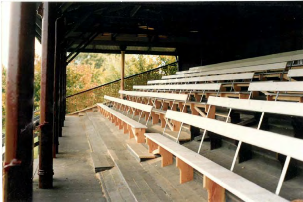
Figure 35 Image of the upper viewing area, looking west, after the reconstruction of the seating and repair of timber flooring and other works undertaken in 1991-92 Source: Courtesy of Terence Nott Architect (copyright Terence Nott)
