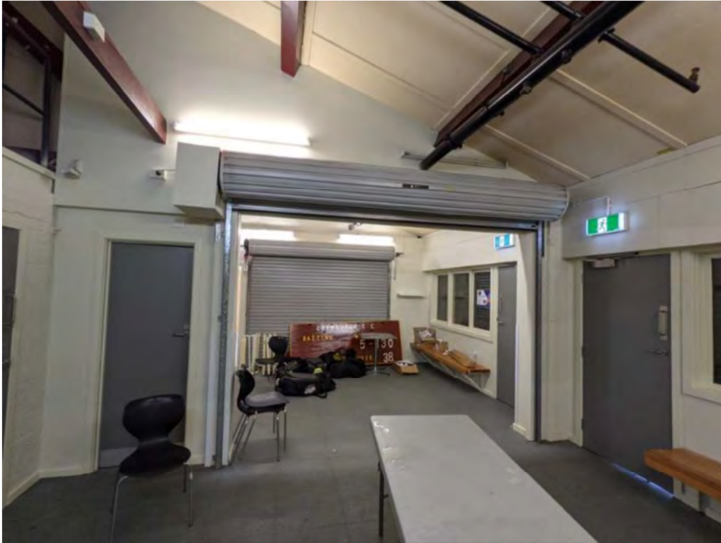
Figure 41 View of the ground floor of the grandstand, looking east; note the modification of the internal walls to create linked internal spaces; mezzanine is visible at left
