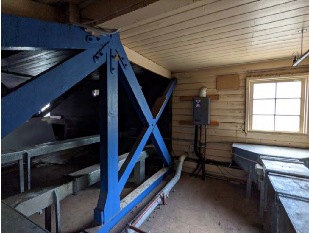
Figure 43 Interior view of the mezzanine area showing timber truss (at left), timber lining boards to wall and ceiling and modern services throughout
