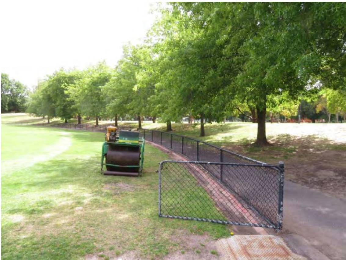
Figure 46 Brick drain, cyclone wire fence and asphalt path to perimeter of oval, with low modern treed berm surrounding.
