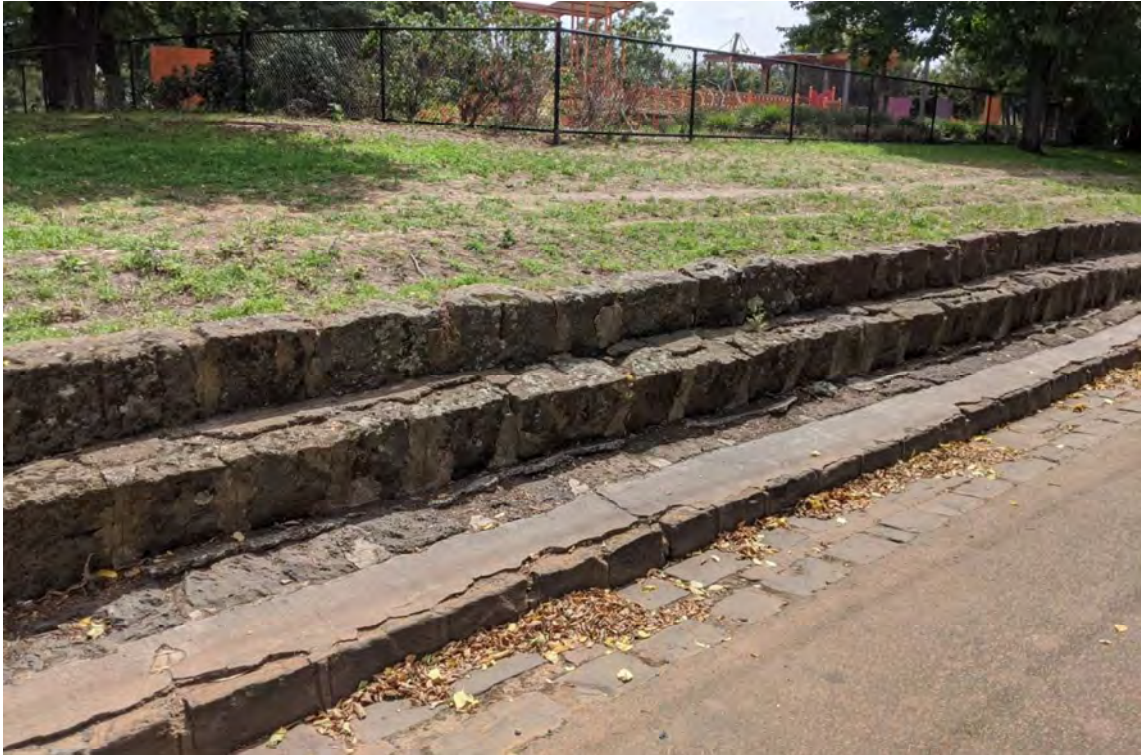
Figure 157 Bluestone retaining wall and gutter along the edge of Alfred Crescent adjacent to the south playground
