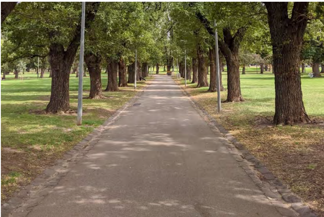
Figure 89 Example of bluestone channel edge without kerbs; similar bluestone channels appear to have been installed in the 1950s-1960s
