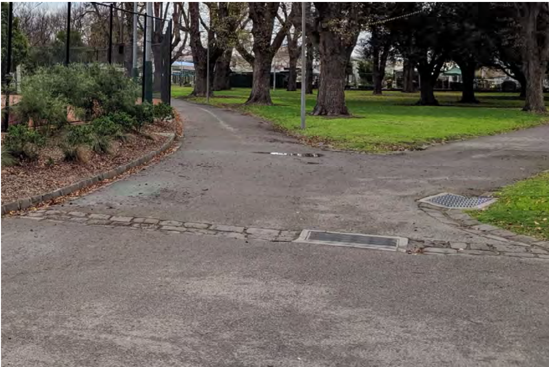
Figure 91 Bluestone channel with later concrete drainage pit at intersection of Avenues A, D and F; aerial photography suggests the channel was installed c. 1950s-1960s
