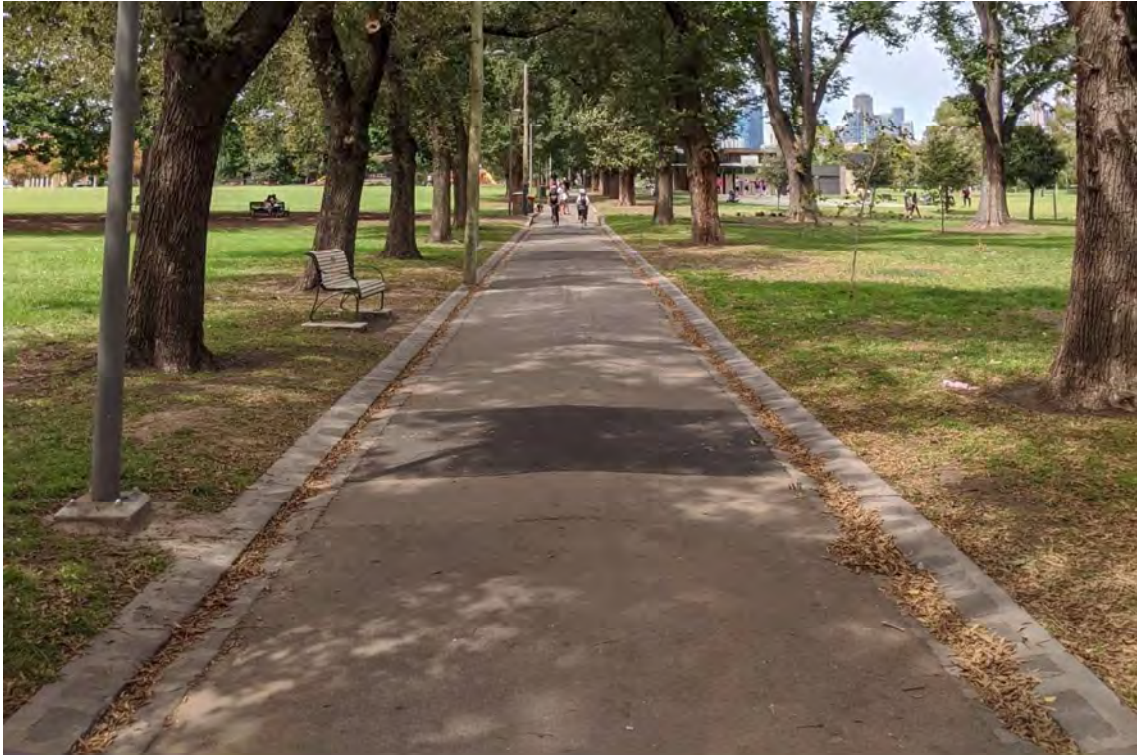
Figure 92 Example of an integrated bluestone kerb and channel, with the outer course raised to form a low kerb above the inner course which serves as the gutter, and heavy concrete mortaring; this edging is likely to date to the c. 1970s
