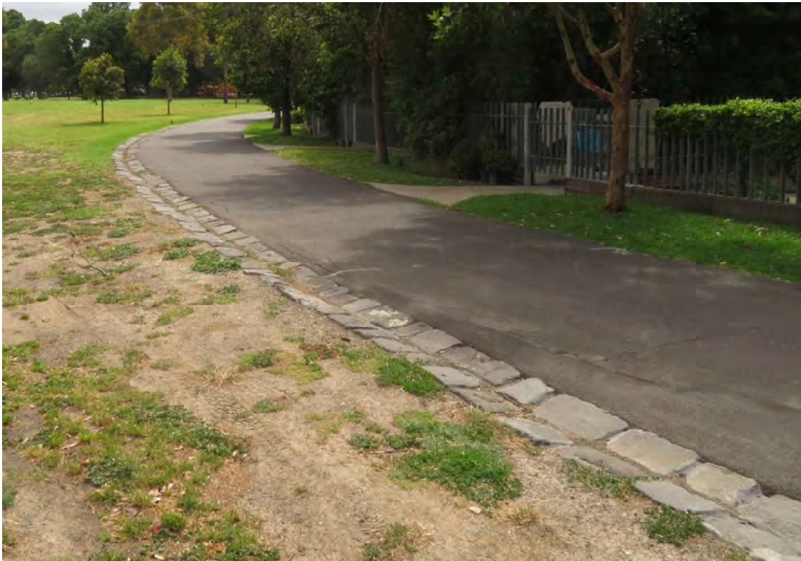
Figure 154 V-shaped bluestone gutter on the path between Alfred Crescent and Freeman Street
