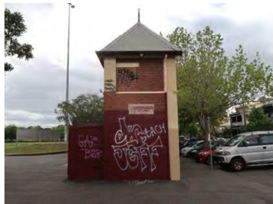
Figure 58 West elevation of the entrance gatehouse; note the former ground level entry has been infilled
