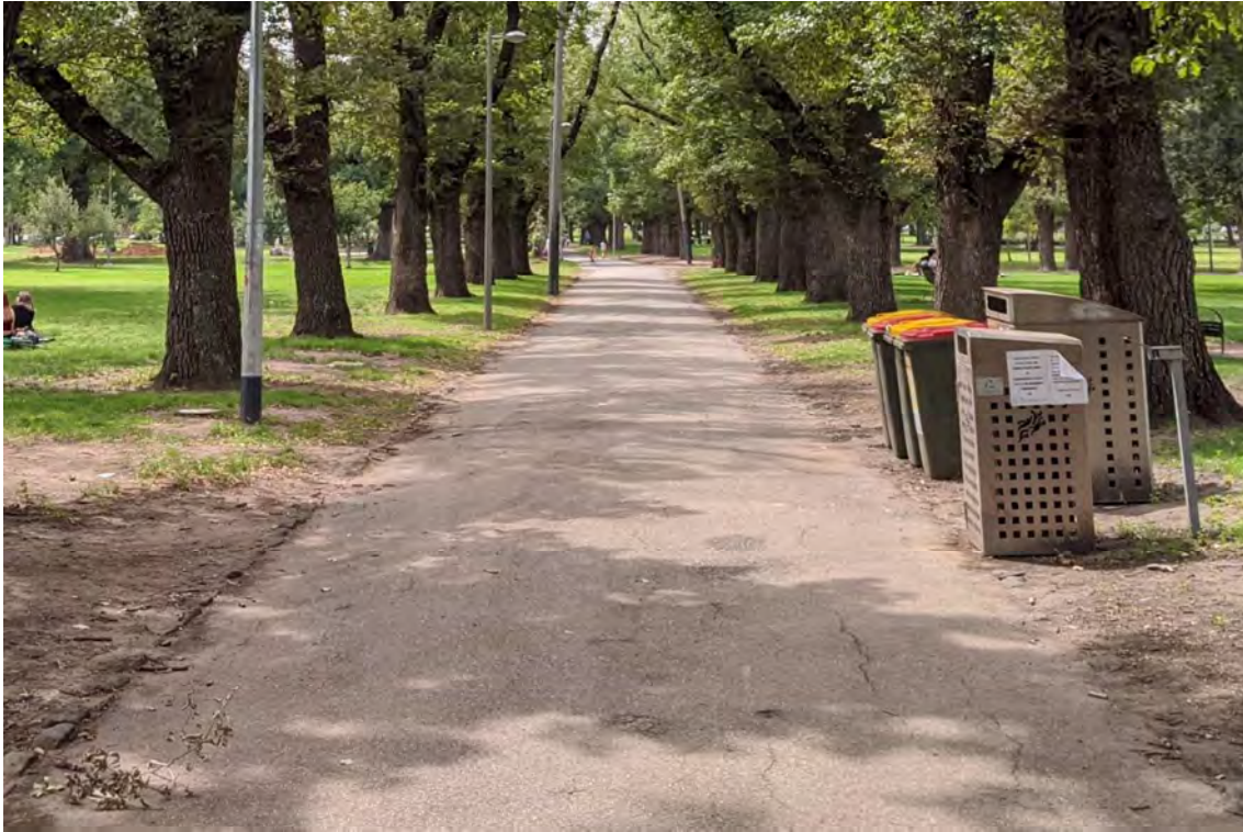
Figure 88 Example of a path with a flush bluestone edge; this edging may have been introduced with modern asphalt paving in the c. 1950s
