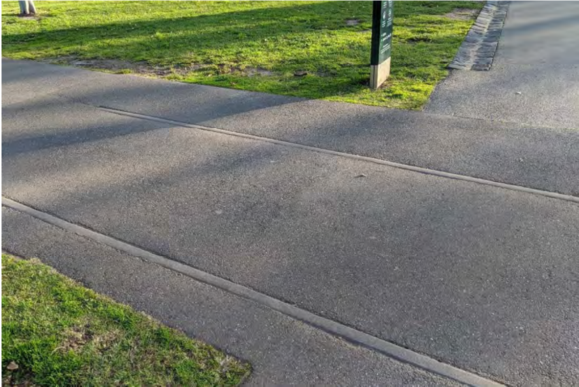
Figure 109 Rails embedded in the pavement of Avenue L in south part of gardens
