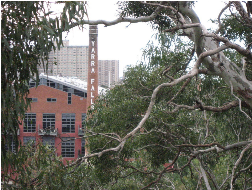
A view of the former Yarra Falls Mills Chimney, 8 Trennery Crescent, view from Dights Falls approx - before development.
