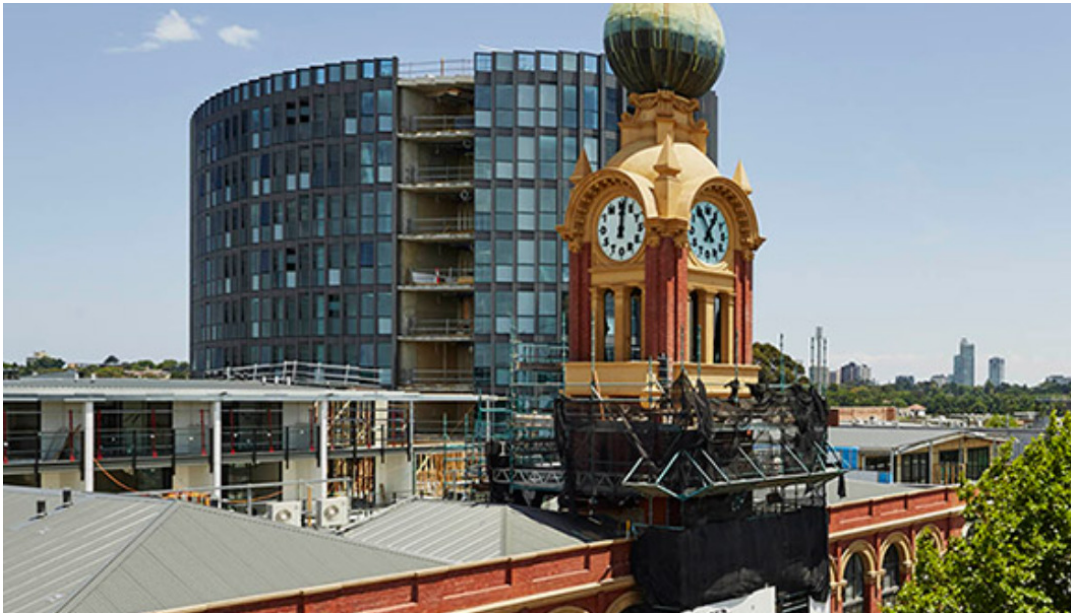
Dimmeys Clock Tower, Elevated View from across Swan St, intersection with Clifton St.
