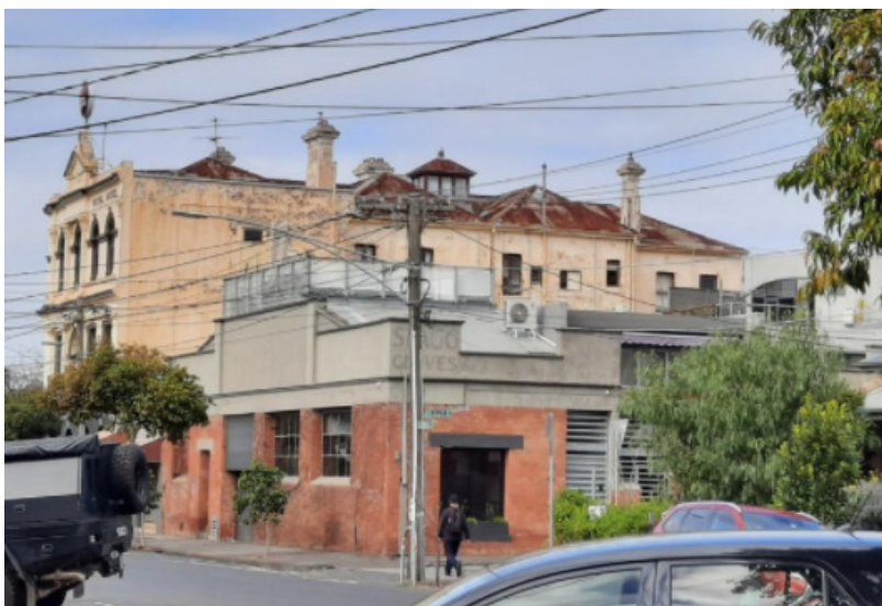
View of Royal Hotel 35-41 Spensley St, from corner of Spensley St and Liley St, Clifton Hill. All the fabric in view except for the facade has been recommended for demolition by Yarra Planning.
